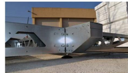
Adjustable support detail.
